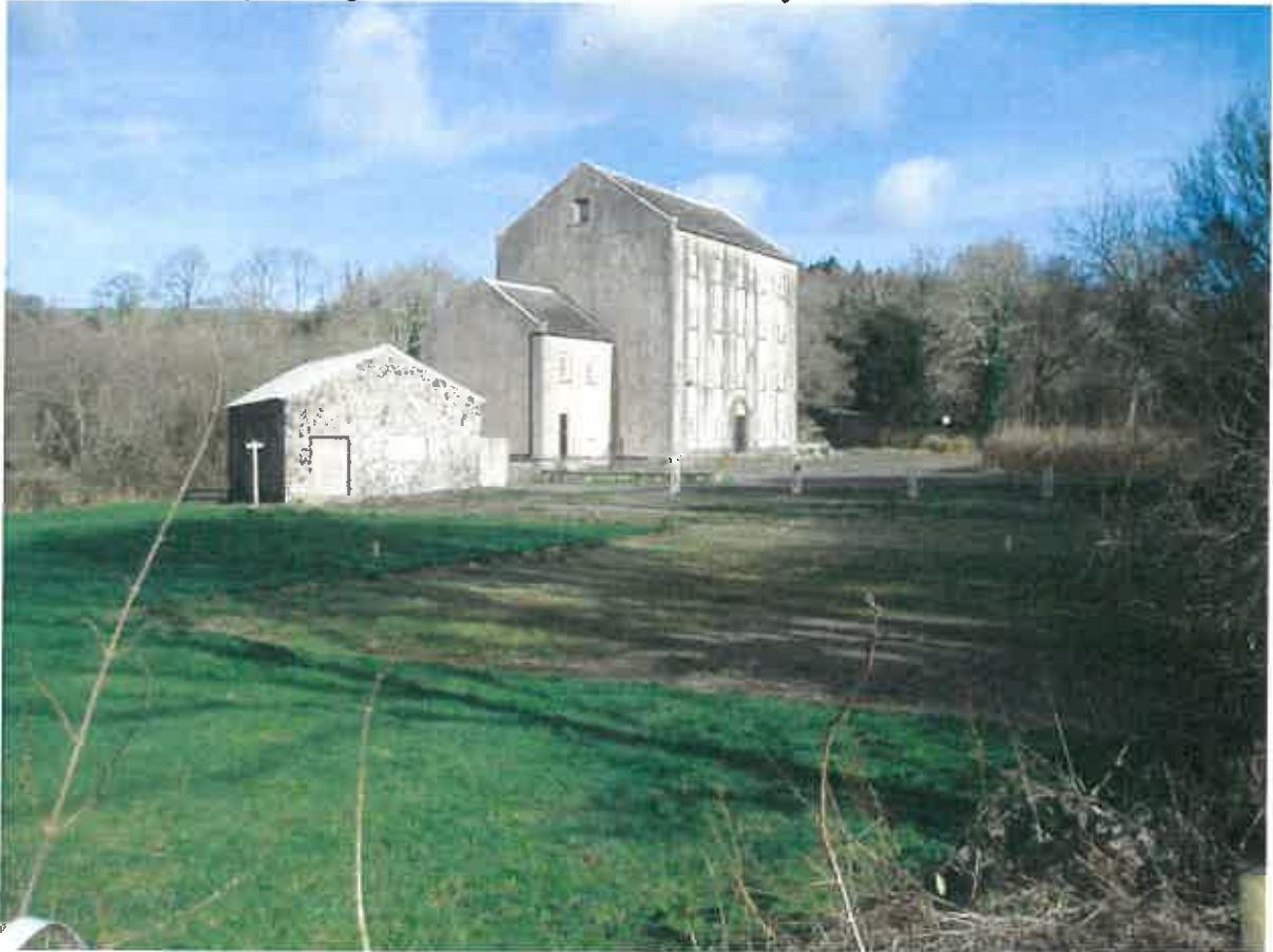
Figure 7 - Mill and former forge building
