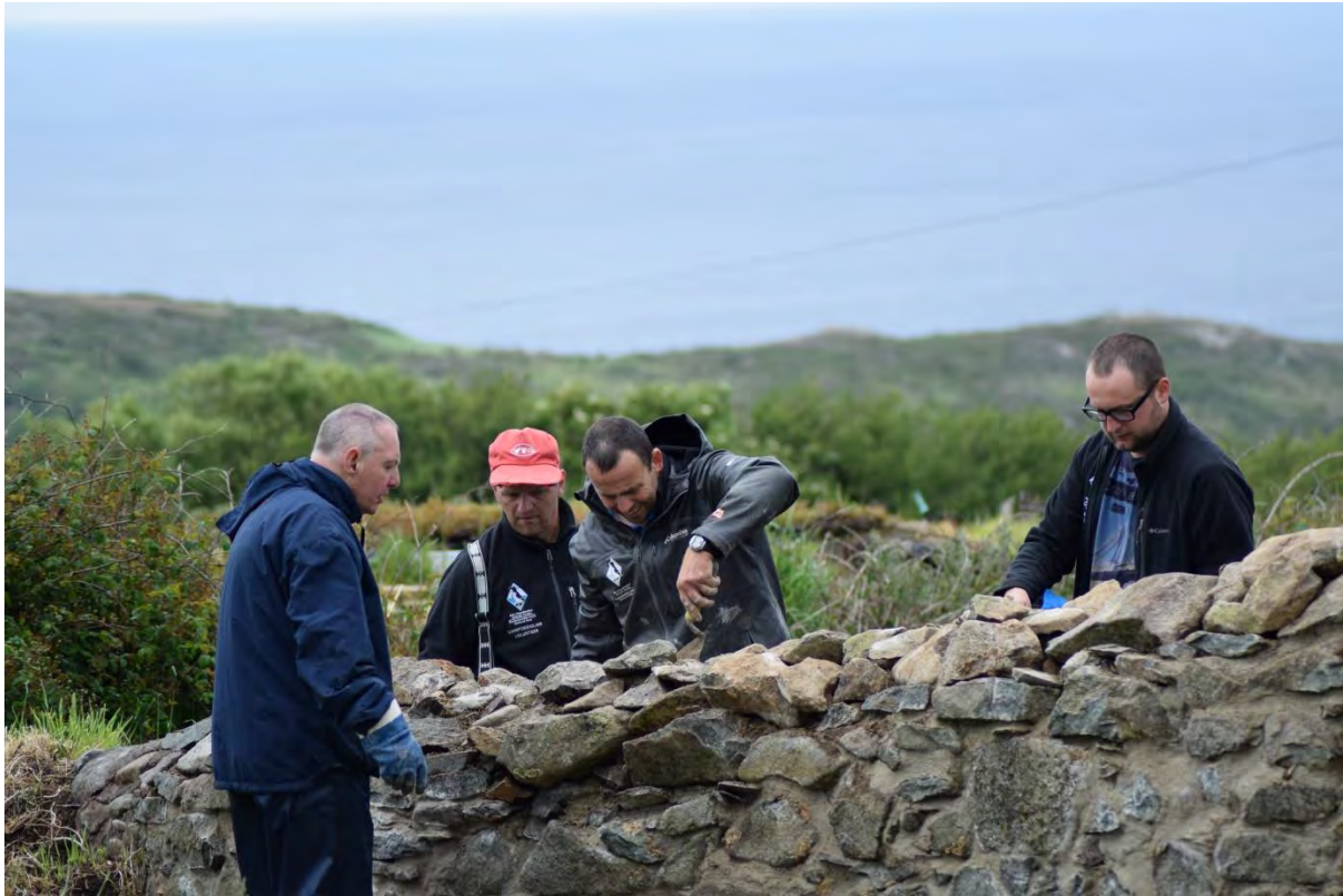
Llanwnda Wall building with volunteers
