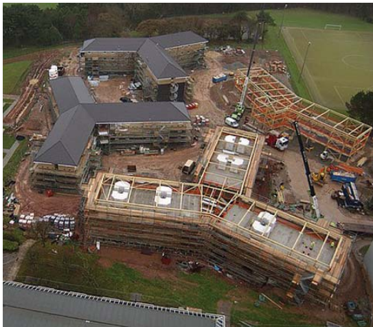
Single Living Accommodation construction, RNAS Culdrose
