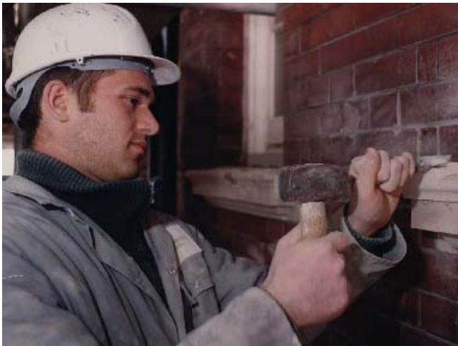
New College refurbishment, RMA Sandhurst
