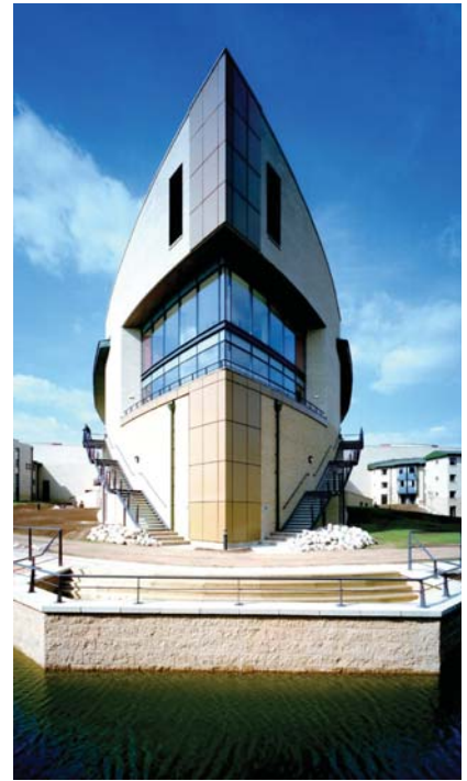
Joint Services Command and Staff College, Shrivenham
