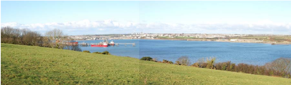
Main channel with jetties in use
