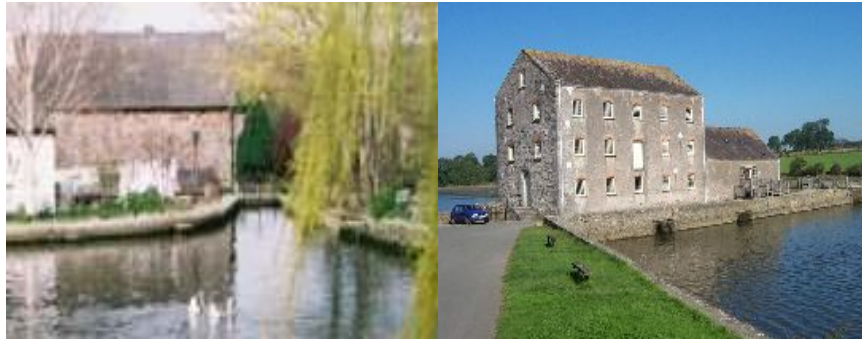
Low head water mill at Y Felin
